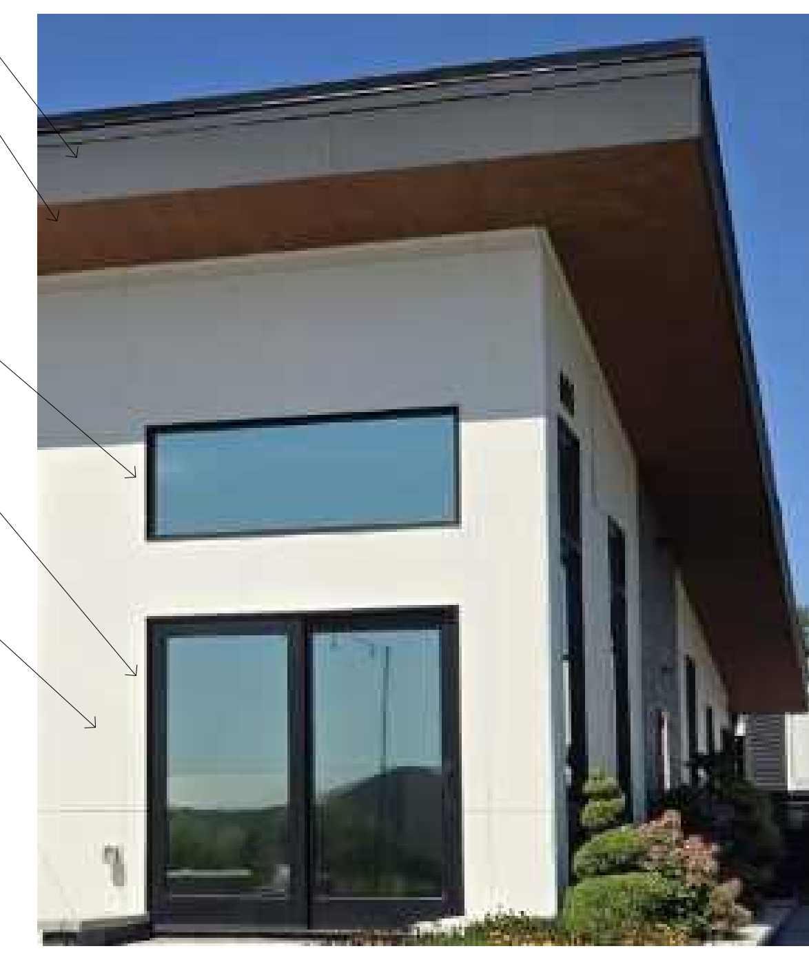
A4 Existing Office Building Photo A102 Not to Scale
