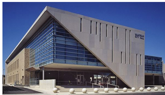
FIGURE 3.9 / WAUKEGAN CITY HALL
