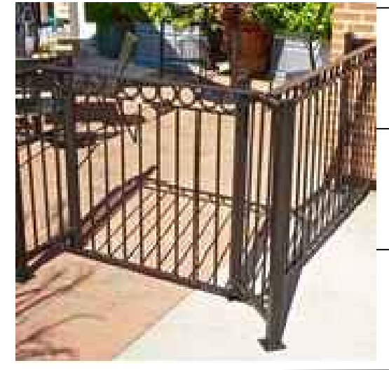
DESIGN INTENT PHOTO: 42" TALL BLACK ORNAMENTAL METAL FENCE AS SHOWN WITH PICKETS 4" O.C. MAX. SPACING, TOP RAIL TO BE FLAT, POSTS TO HAVE POST CAPS. FENCE TO BE CONTINUOUS AS SHOWN.
