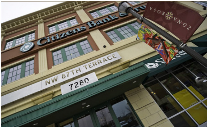
Multi-Tenant Wall Signage Vertical
