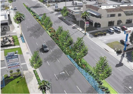
New median to limit roadway cross-access
